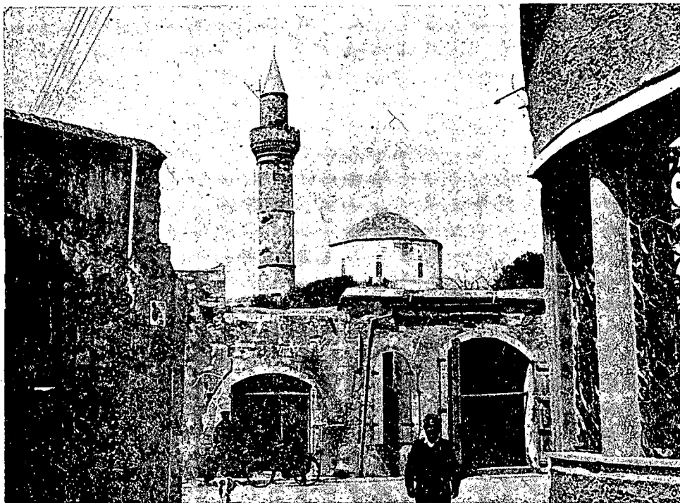
Minaret O.P., Ktima seen from the Green Line.
