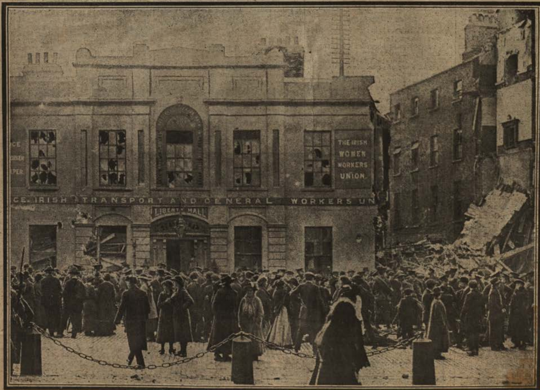
Ruins of Liberty Hall, the rebels' headquarters, which was shelled by a gunboat from the Liffey.
