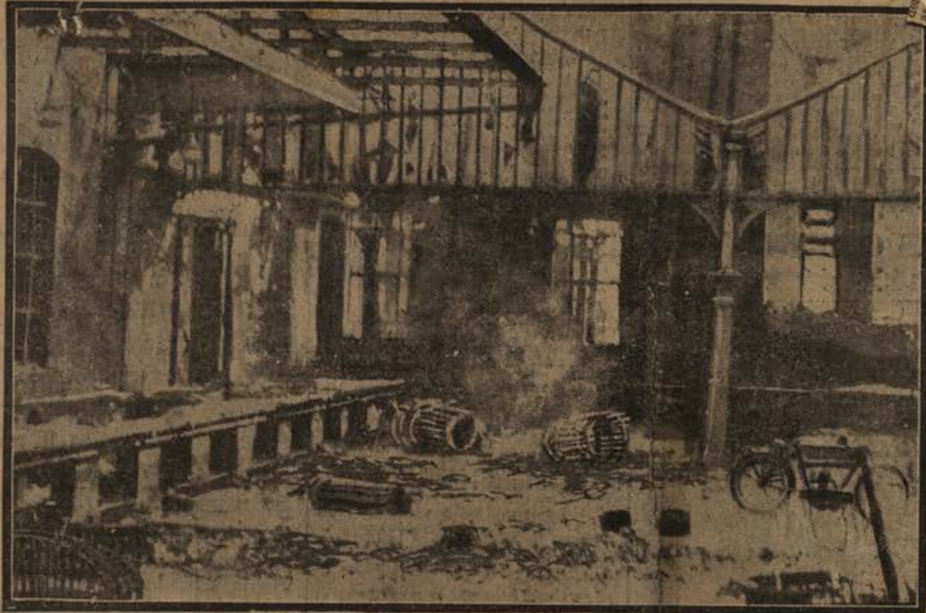
INSIDE THE POST OFFICE. —"Fighting raged through the ground floor of the great building, which, after wild and furious resistance, was eventually cleared of the rebels at the point of the bayonet." This photograph shows part of the still smoking interior of the building after the rebels had been driven out. ["Daily Mail" Photograph.]
