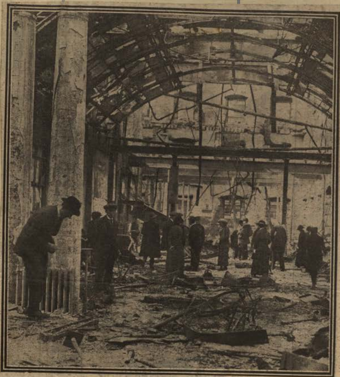
Inside the Post Office, which has been reduced to a four-walled, roofless shell.
