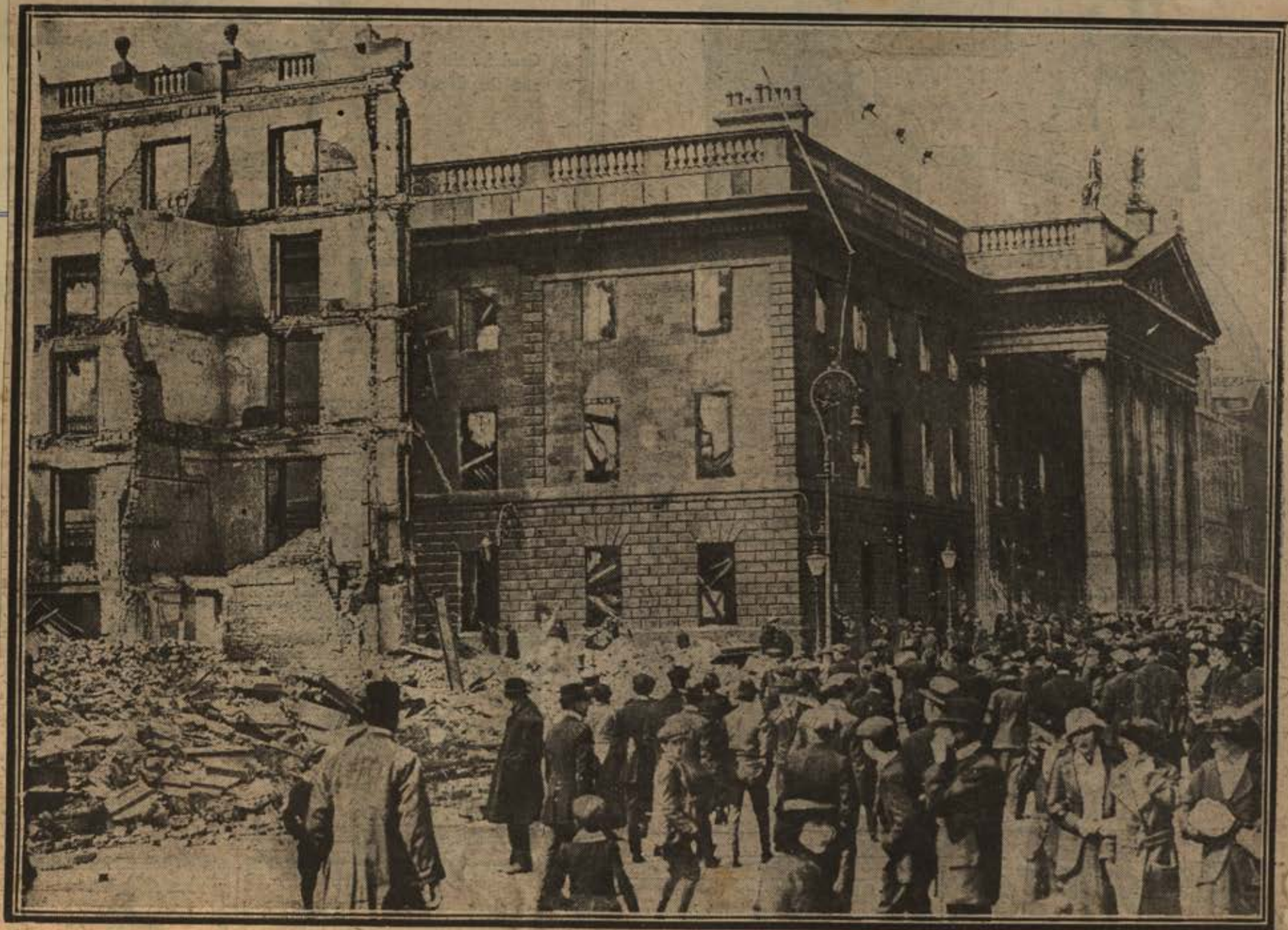
West side of Sackville-street, showing ruins, and the General Post Office, which was seized by the rebels.
