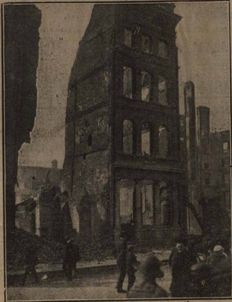
All that remains of the English and Scottish Law Life Assurance Buildings, of Messrs. David Drimmie and Sons', at 41 Lower Sackville street. The vacant space to the right was formerly the shop and library of Messrs. Eason and Son, Ltd.
