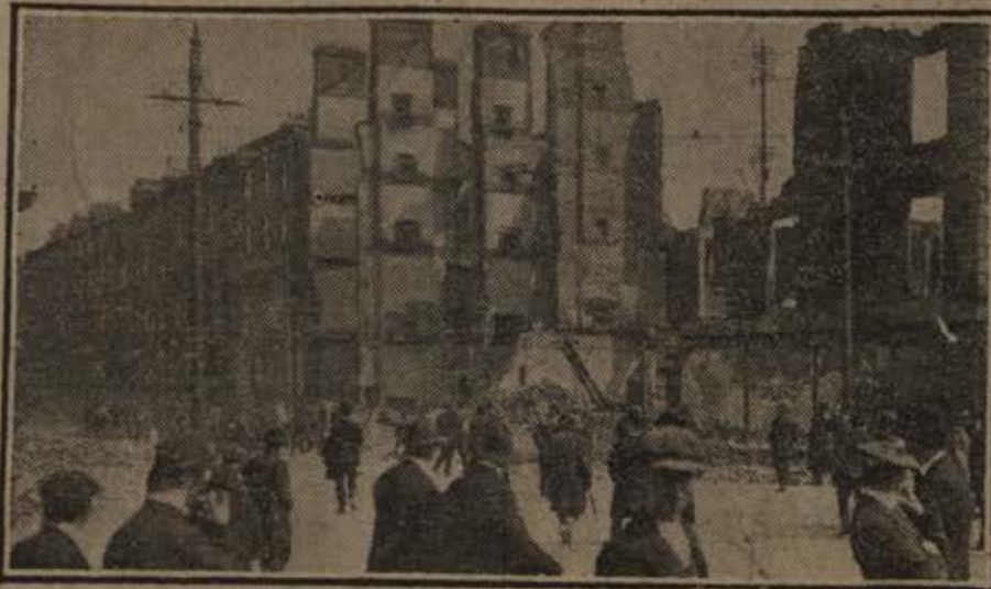
Lower Abbey street, as it appears from where the Hibernian Bank Branch Office stood. The premises destroyed include the Royal Hibernian Academy, Wynn's Hotel, Messrs. Smyth and Co., hosiers; J. Ferguson and Co., hair-dressers; and Charles L. Reis and Co., jewellers.
